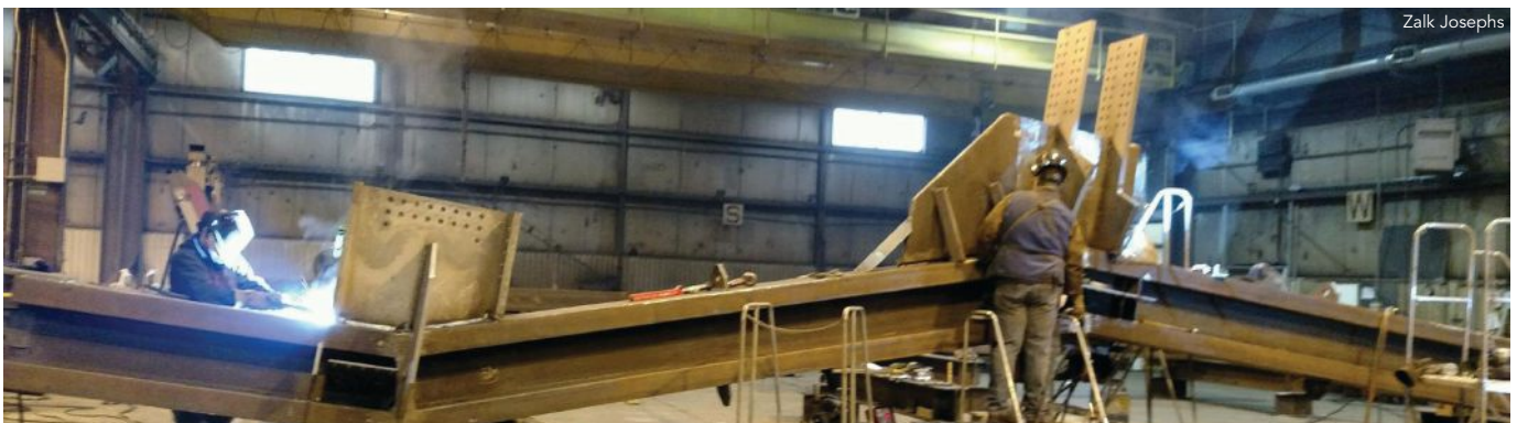
below: Assembling kinked columns at Zalk Josephs' fabrication shop.
